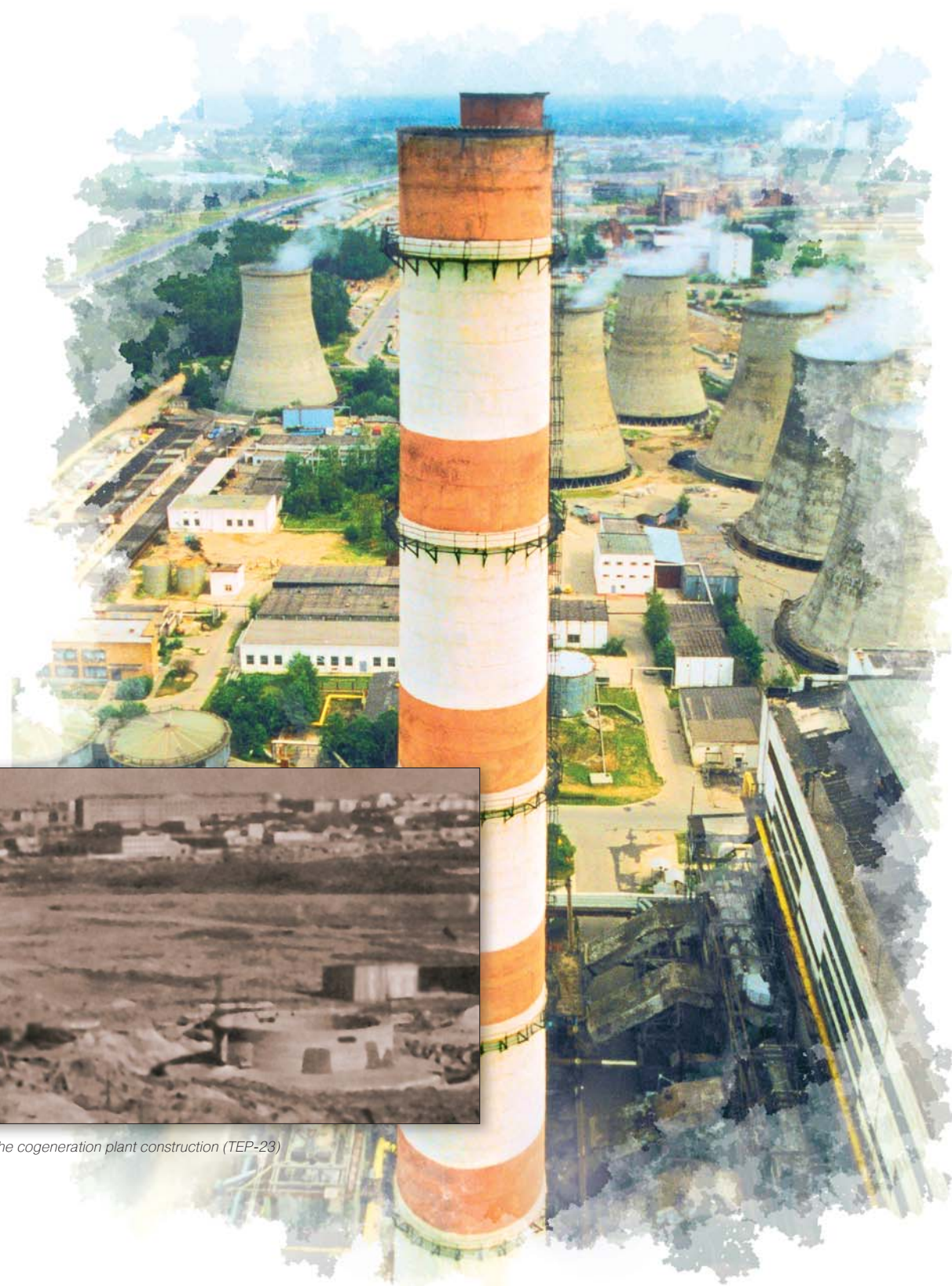
2002. Cogeneration plant today (TEP-21)
