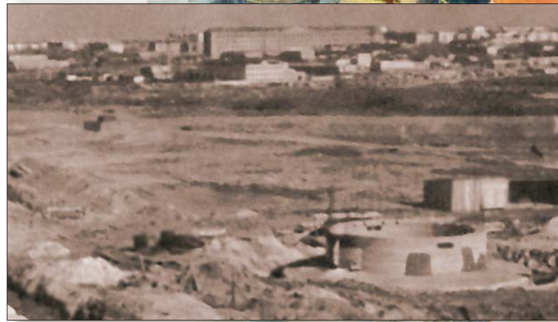
1960's. Beginning of the cogeneration plant construction (TEP-23)
