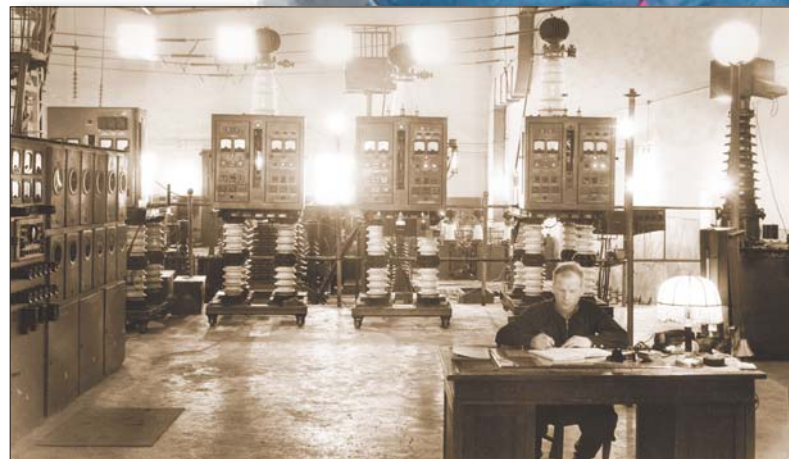
1956. Process monitoring at the substation
