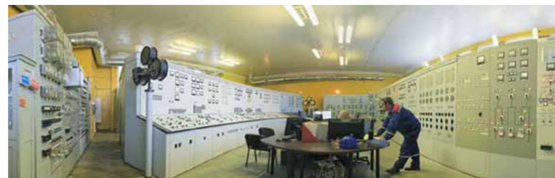
Fig. 66. Main control room at Svetogorskaya HPP
