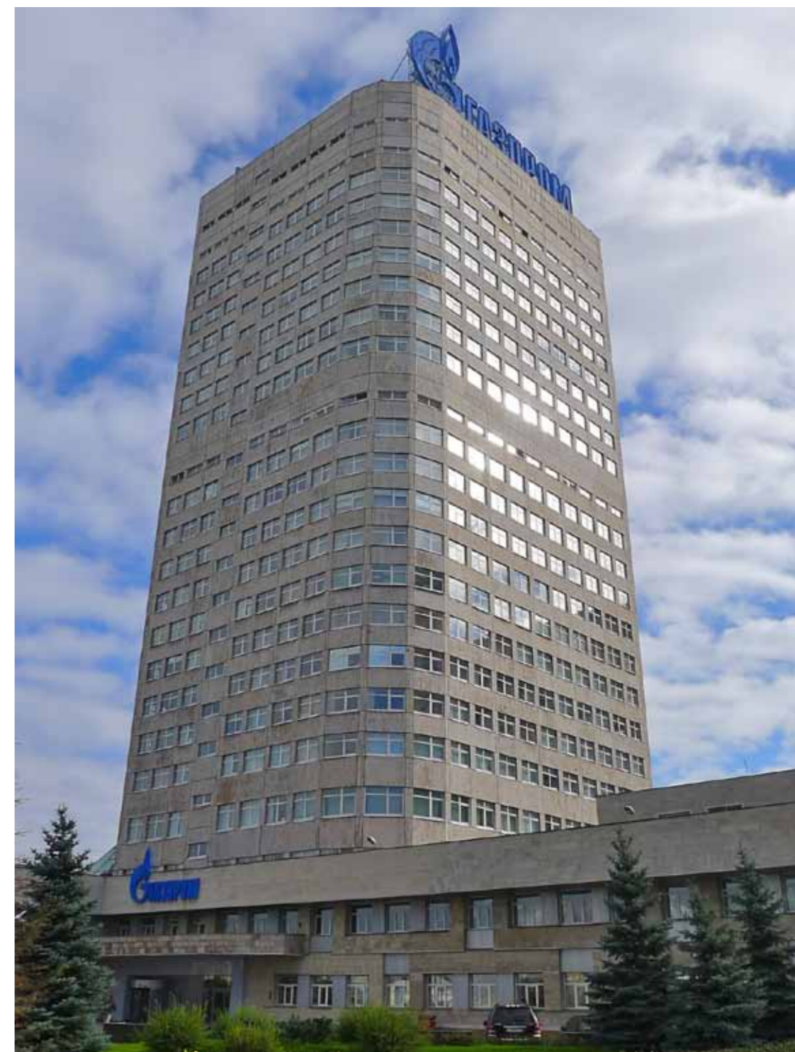
Fig. 1. OOO Gazprom Energoholding, OAO Mosenergo, OAO OGK-2 headquarters, Moscow
